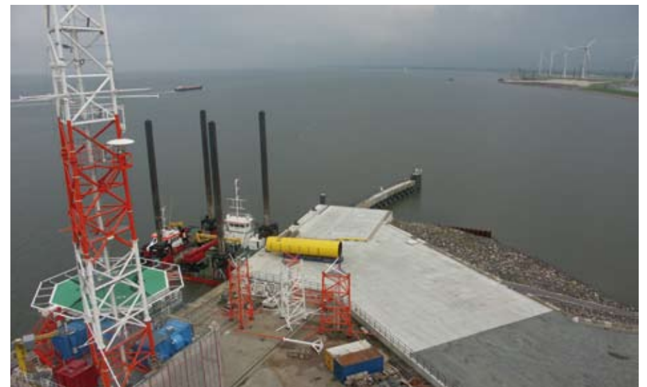
Heavy load platform of the OffshoreBase Cuxhaven.
